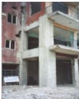
Retrofit of apartment building in Gulcuk
