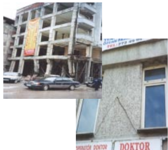
Damage to buildings in Adapazari
